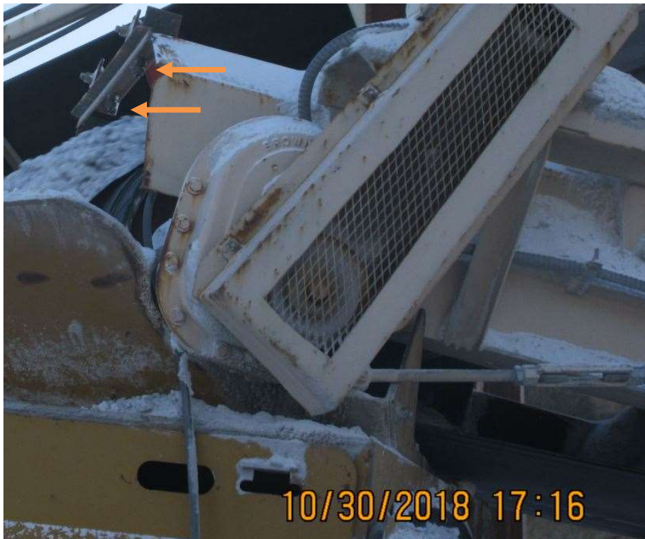
Photo 2- Water Sprays Not Operating
