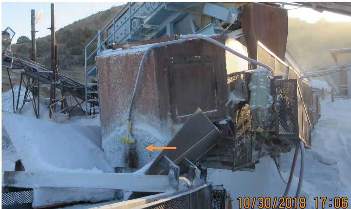
Photo 4 – Spray has not Been Formed Over the Area Where Particulates are Emitted From
